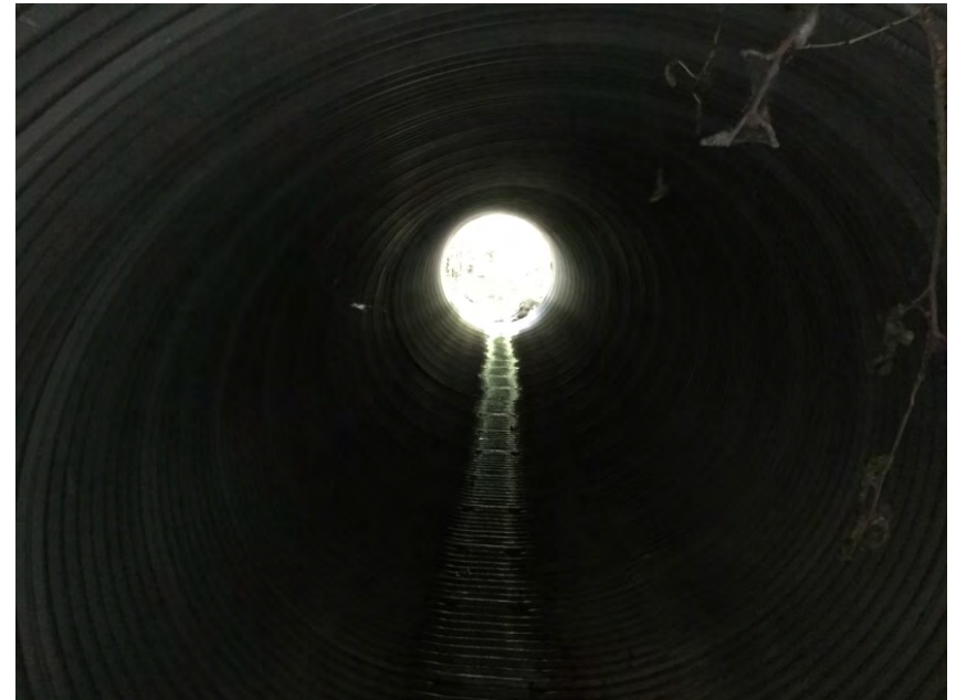
Looking through from inlet
