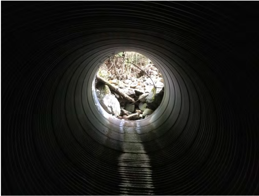
Material building up at inlet
